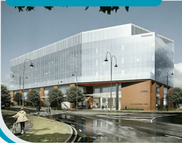
MUNROE LANE OFFICE BUILDING - NZ
